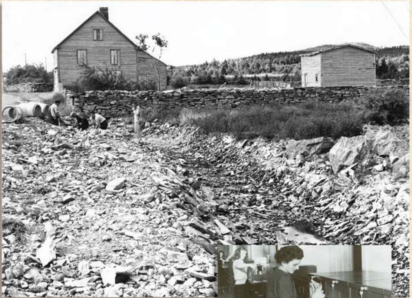
6.50 Constructing a sewer pipe
